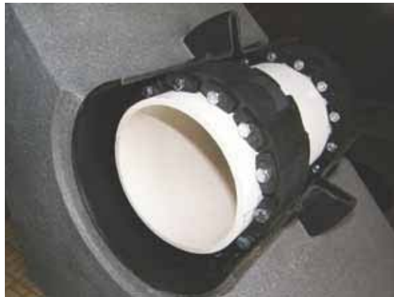
Cut-away view of Infinity® wall sleeve & Innerlynx®
