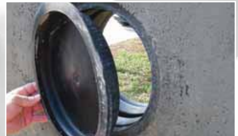
6. After concrete is cured, pry off the locator caps with a pry bar.
