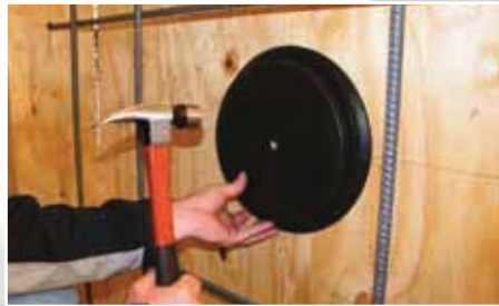
2. Screw or nail one of the locator caps at the center line.
