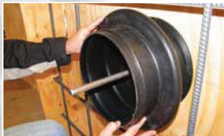
2. Attach Infinity® wall sleeve to locator cap.
