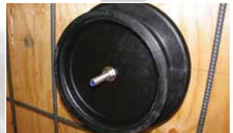
3. Slide second locator cap through (threaded rod*), use fender washer and fasten nut until locator caps and sleeve are locked in place. Check to make sure sleeve is square to form.
