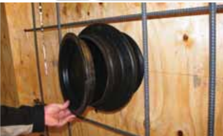
4. Insert the second locator cap.
